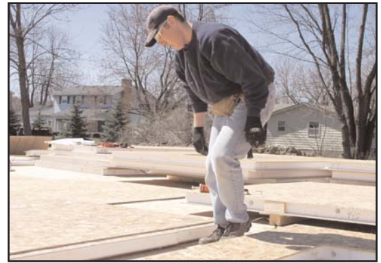
SIP panels are numbered and have precut wire chases to expedite the building process.
