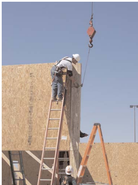
PorterSIPs panels are nailed into place at the Holland, MI O'Charley's Restaurant
