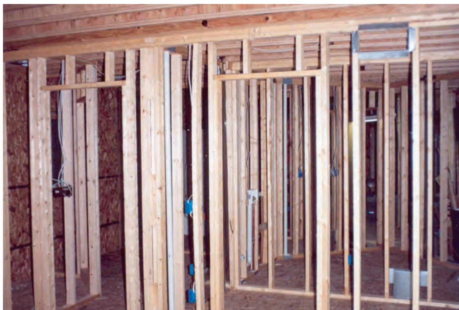
HVAC ducts are placed in the stick-built parts of the PorterSIPs home
